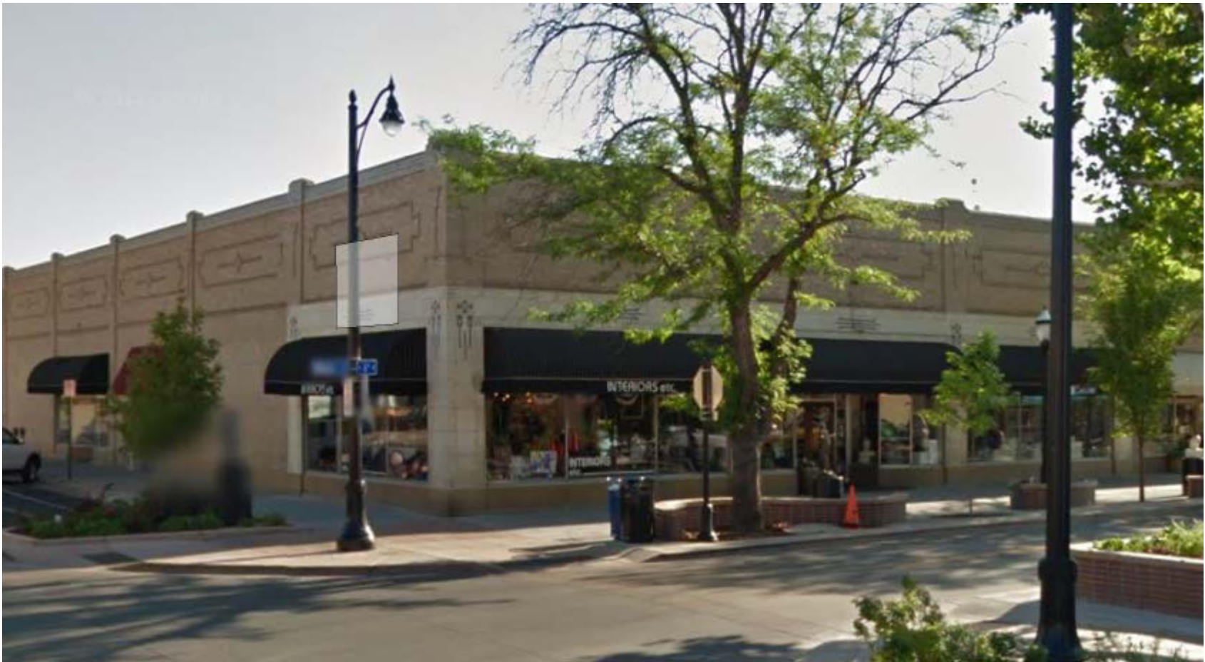
602 Main Street Current Google Street View July 2012
