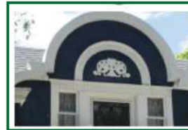
Example of a Parapet
