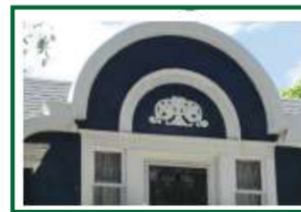
Example of a Parapet
