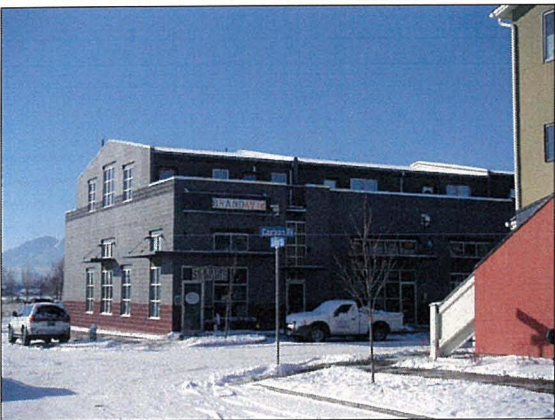
Third story is stepped back from the street edge to minimize massing as perceived from the street. (Boulder, CO)
