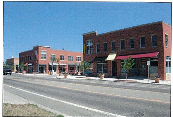
Architectural detailing includes increased massing at the street corners. (Boulder, CO)
