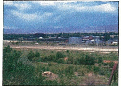
Tanks of the Koch Plant
