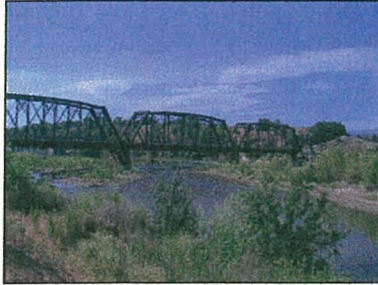
Railroad bridge at the south end of the site.
