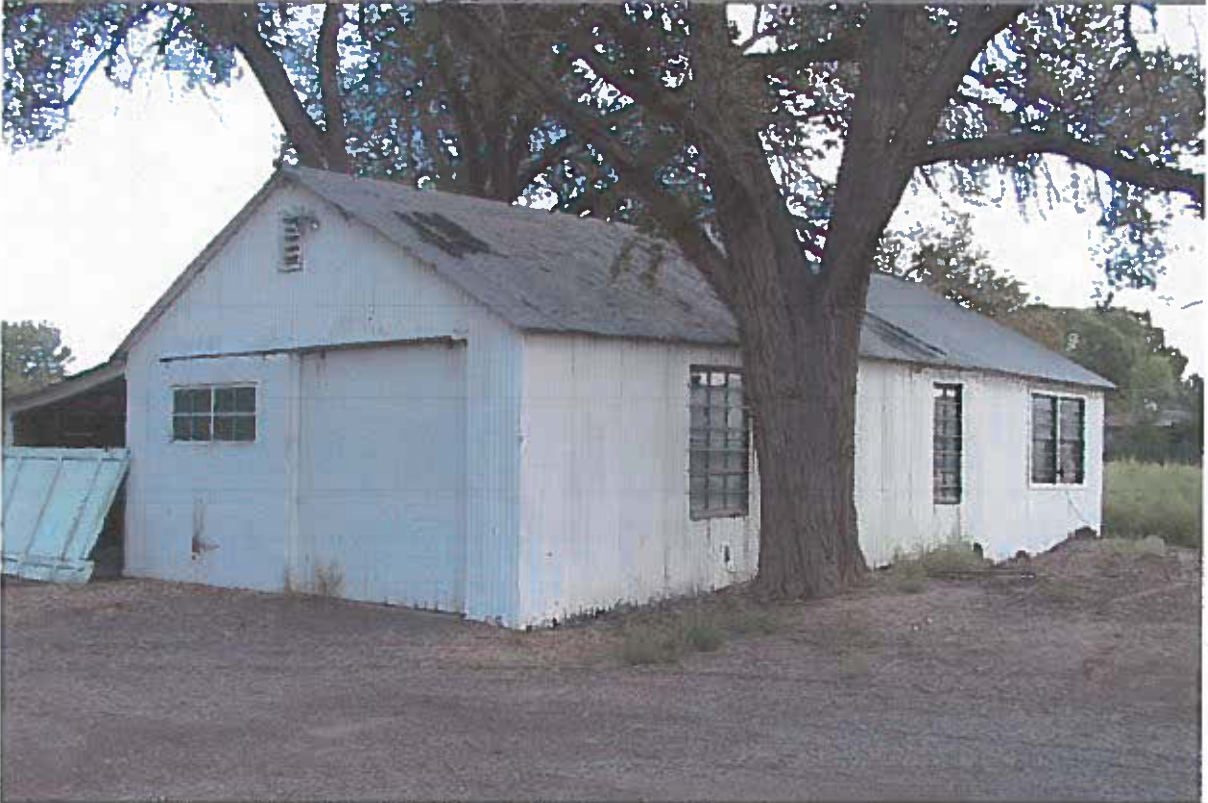
EXISTING GARAGE – 276 Linden Avenue CDBG 2003-08 City of Grand Junction
