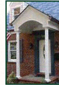
Example of a Portico
