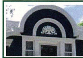
Example of a Parapet
