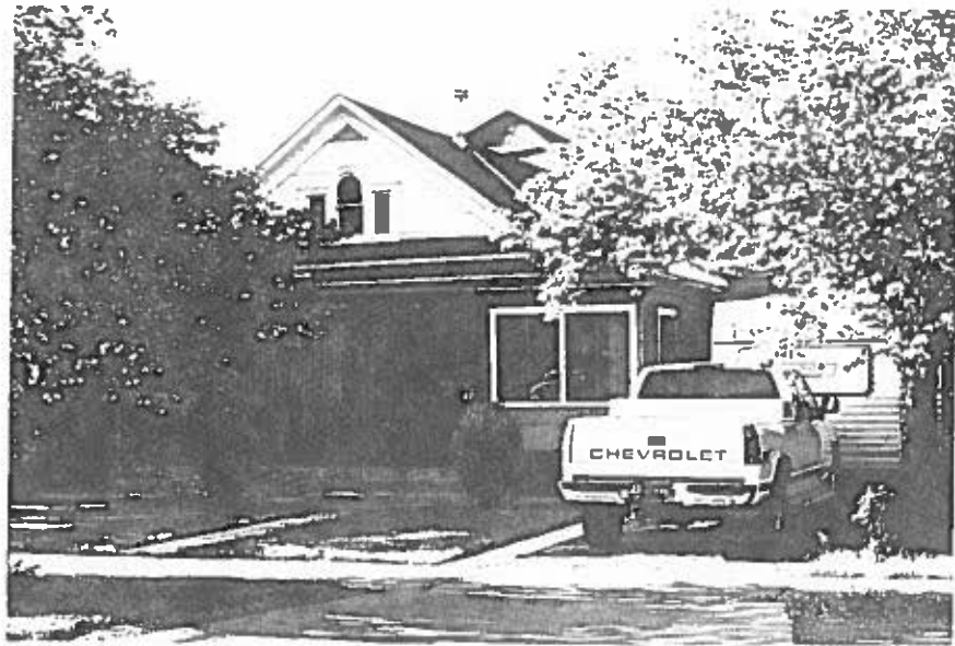
747 Colorado Ave. , Grand Junction, Mesa Co, CO 2945-144-29-010 05/14/1996 Roll 44 Frame 24 View N Dir SE 5ME8568
