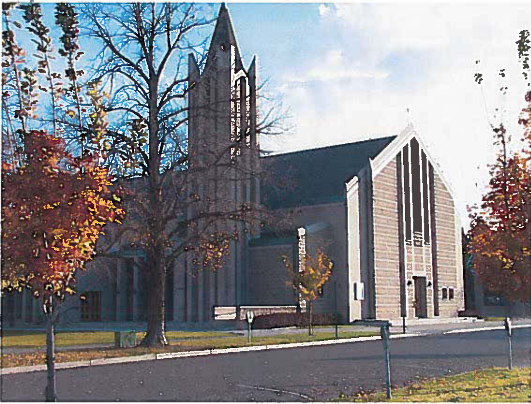
St. Joseph Catholic Church, Grand Junction (new, current) From southwest, constructed 1993
