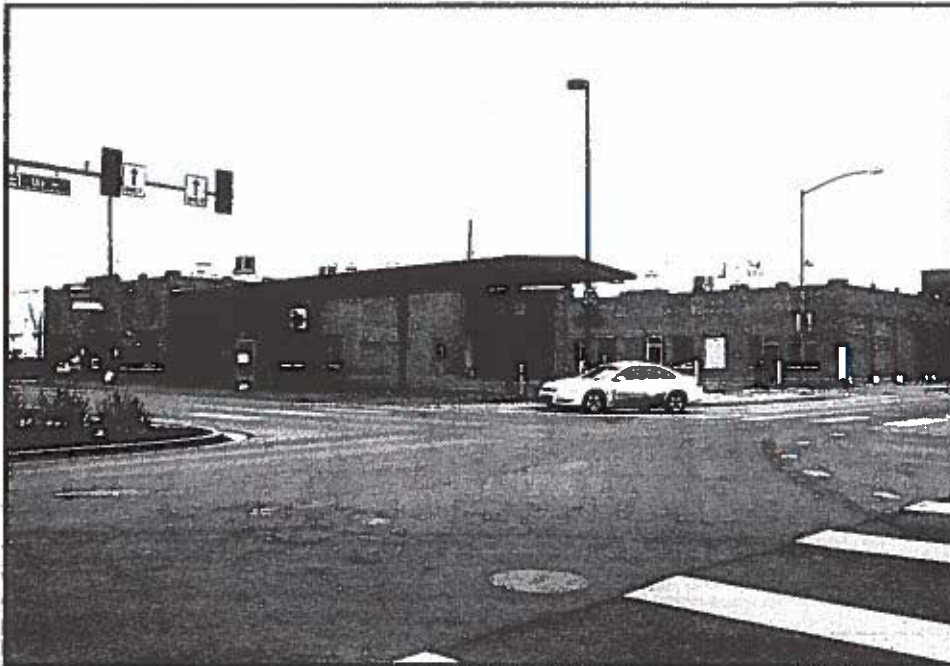
View to Northeast
