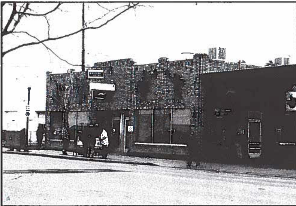
View to Northeast
