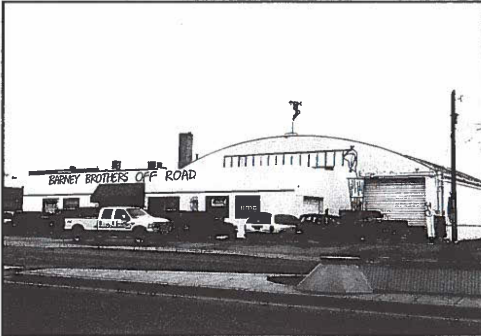
View to Northeast
