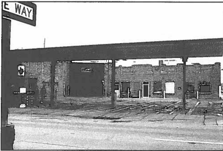
View to Northeast
