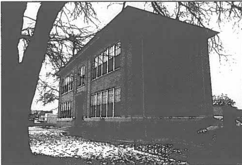
View to Northeast
