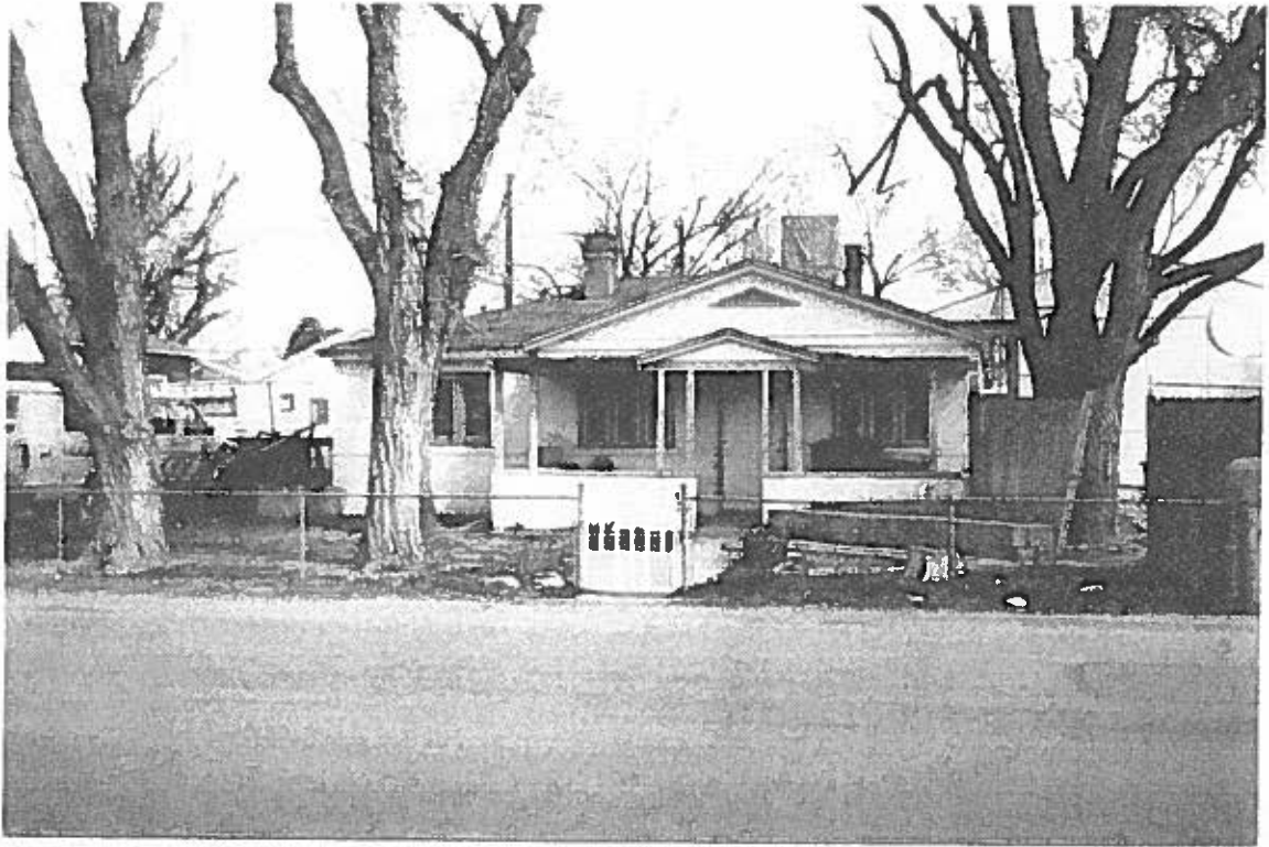
House - View to East
