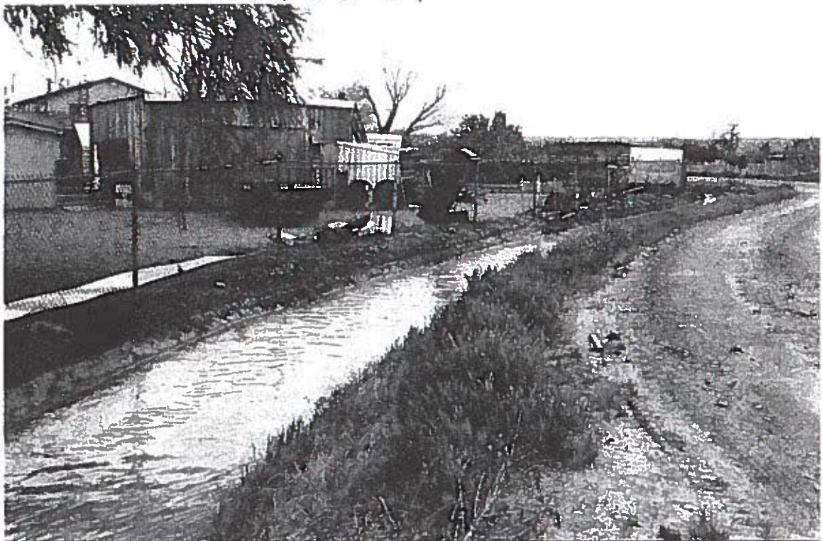
On east side of 29 Road - View to southeast with water in ditch
