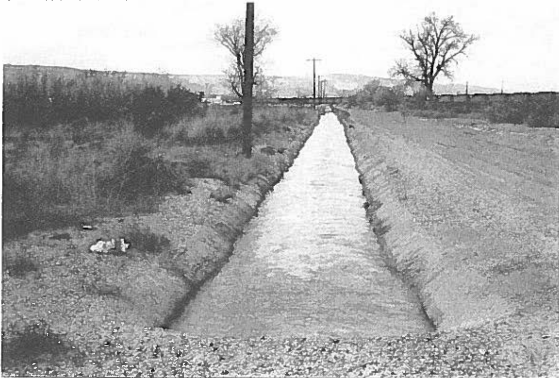
On west side of 29 Road - View to west
