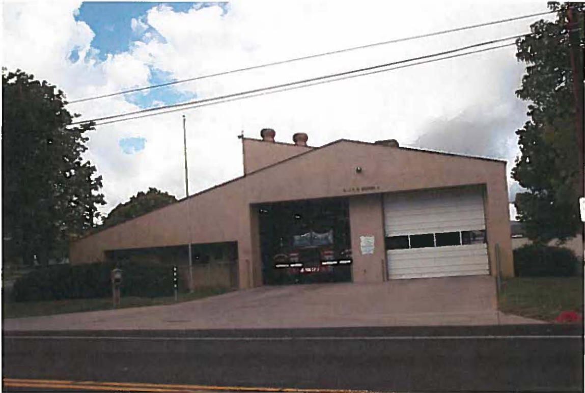
VIEW EAST SIDE BUILDING: FROM EAST TOWARD WEST
