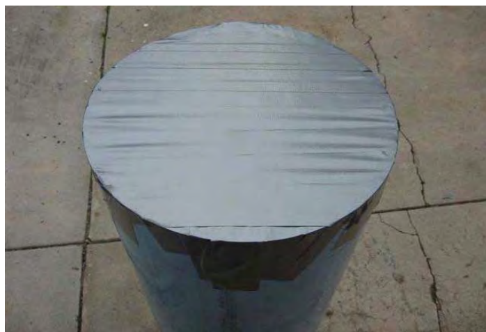
Figure 2.4.2 – Sealing of Pipe End Prior to Pull Head Installation
