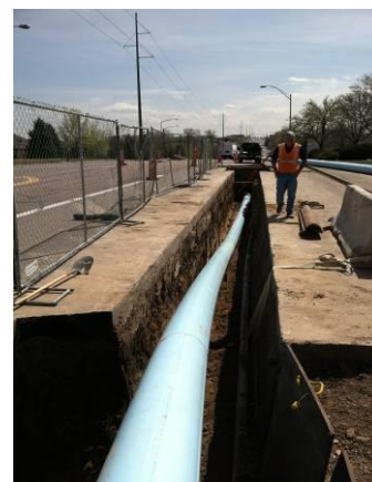
Pipe Insertion – Facing South
