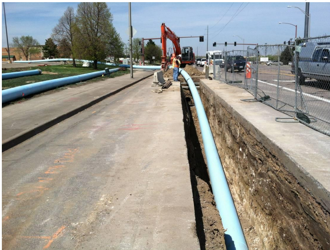
Pipe Entrance Pit – Facing North
