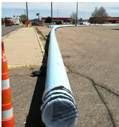
Fused Pipe String
