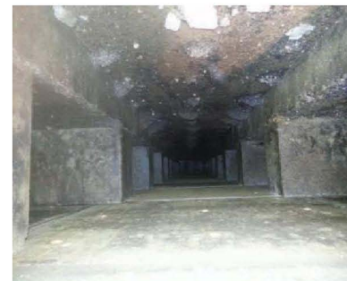
Wheeler Underdrain False Bottom
