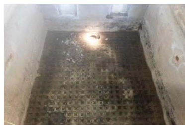
Wheeler Filter Underdrain
