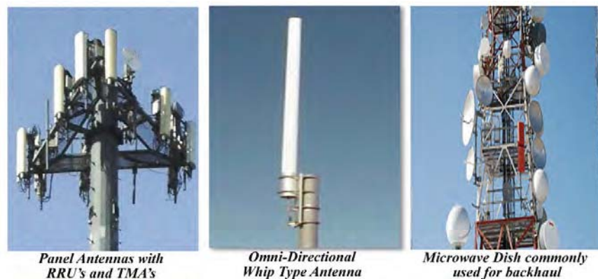
Figure 3: Examples of Panel, Directional and Microwave Antennas
