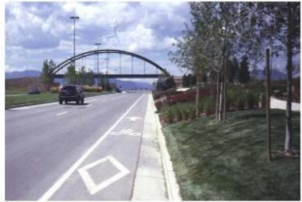
On-street bicycle route designation separate from the roadway
