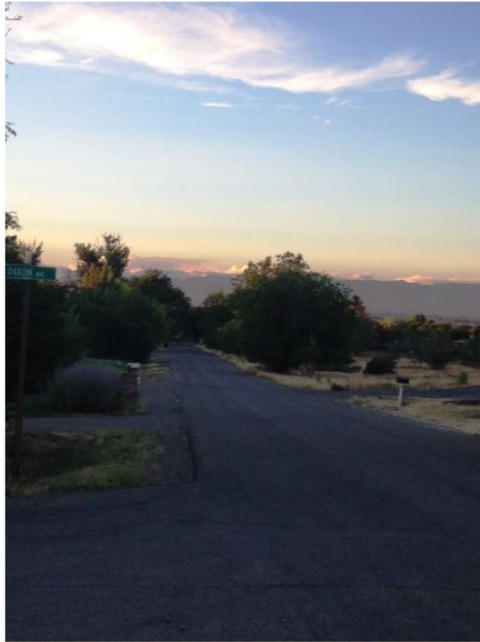
View from the corner of Dixon and 22 ¼ Road, facing northeast towards the proposed subdivision, which can be seen to the right. There is no shoulder, minimal ditching, no lines, rough paved surface, and no turn around (the road dead ends at the canal). This would be the only access to the proposed subdivision and no road improvements have been planned.
