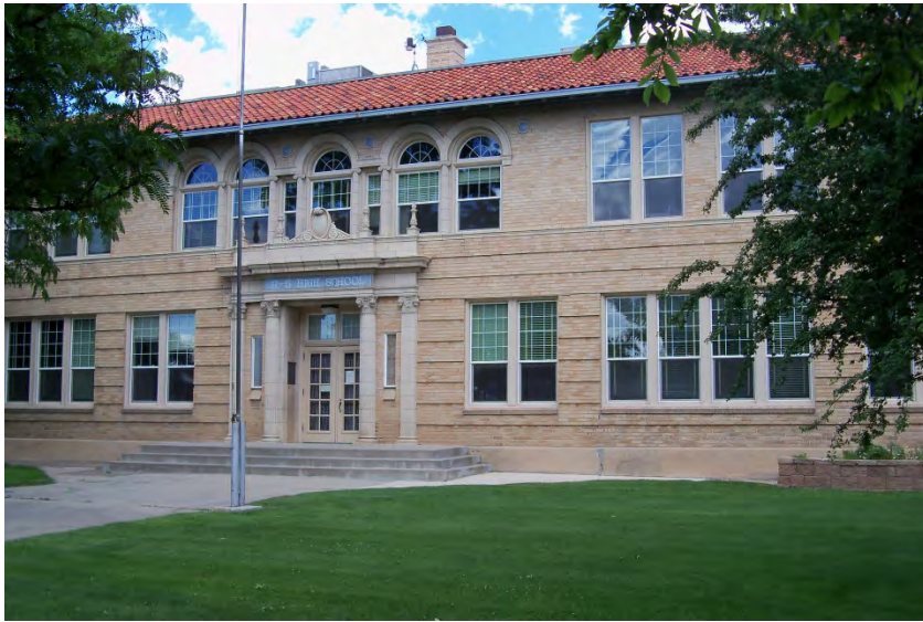
Front of building looking east
