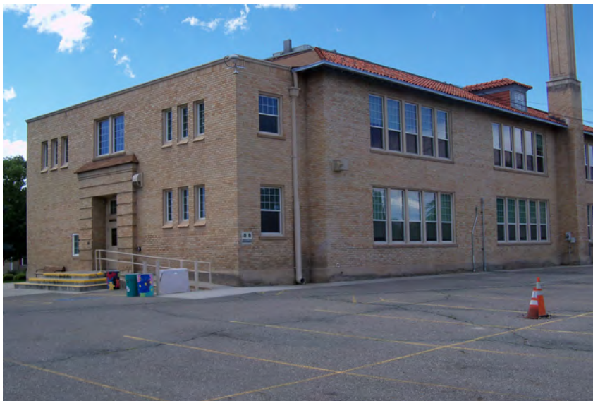
Back of building looking southwest
