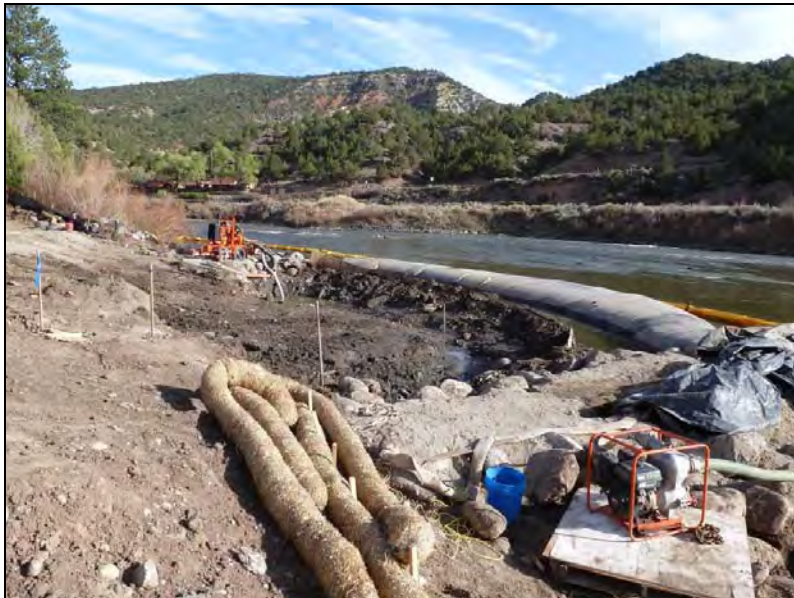
Example of dewatering.
