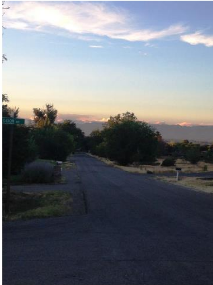
View from the corner of Dixon and 22 1/4 Road, facing northeast towards the proposed subdivision, which can be seen to the right. There is no shoulder, minimal ditching, no lines, rough paved surface, and no turn around (the road dead ends at the canal). This would be the only access to the proposed subdivision and no road improvements have been planned.
