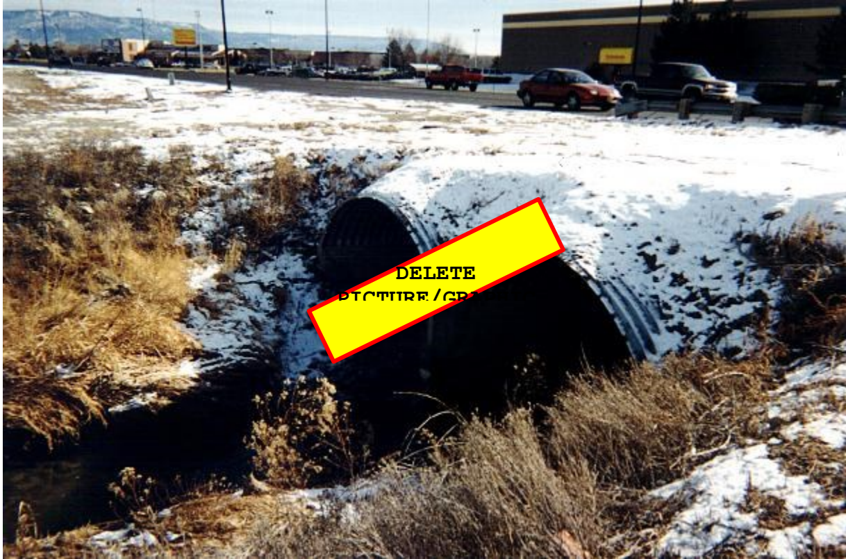
Existing Leach Creek drainage structure along 24 Road
