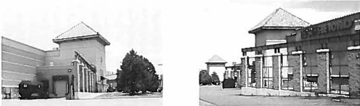
Screening blocks views of loading and storage areas
