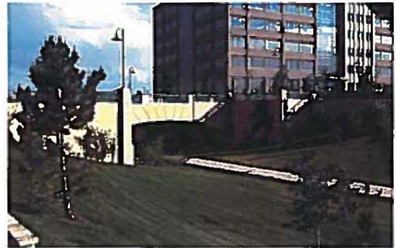
Open space incorporates drainage facility and amenities
