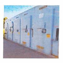
**Description:** The Persigo Treatment Facility has an incoming power supply of 1,302 volts. Power enters the treatment facility through a main control panel which can be used to disconnect power from entering the treatment plant to facilitate repairs.
