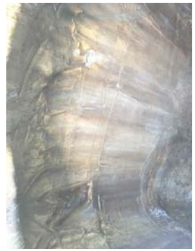
WET WELL NO. 2
