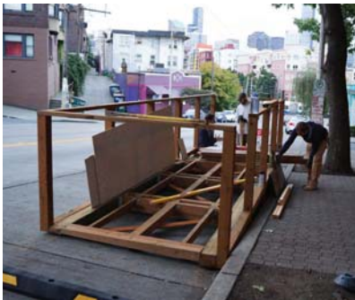
Wood-frame construction of Parklet
