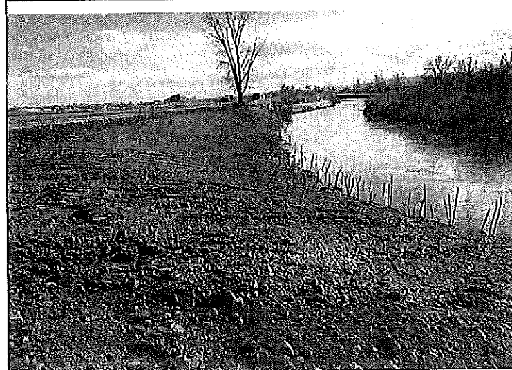
3 Job | Bellvue Water Treatment Plant - River Restoration Contact | Dan Moore (City of Greeley)
