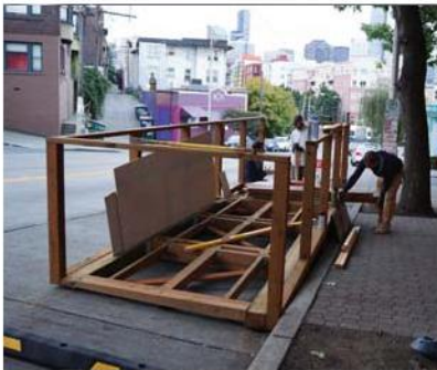
Wood-frame construction of Parklet
