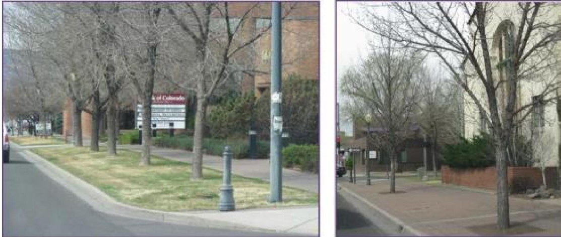
Existing Grand Avenue Streetscape
