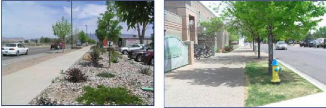
Existing Detached Sidewalk on Riverside Parkway (left) and South Avenue (right)
