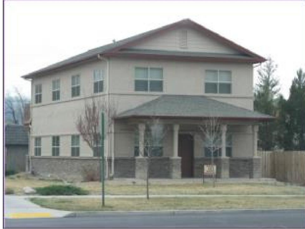
Example Infill Development in Transitional Area - 9 th Street and Colorado Avenue
