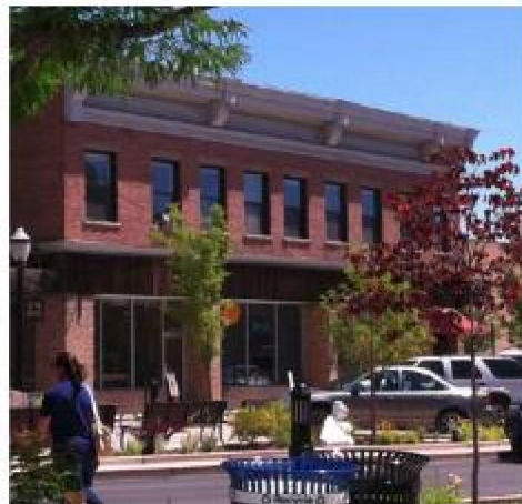
Existing facade with Diminishing Fenestration on Upper Floors
