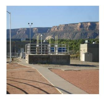
**Description:** Diversion Structure #3 is designed to direct flow to the final clarification process. This process is one of the final stages of treatment prior to discharging water to the Colorado River.
