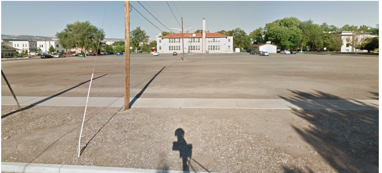
R-5 High School Site Looking West Platted Alley to be Vacated is Undeveloped but Building was Constructed Upon Right-of-Way
