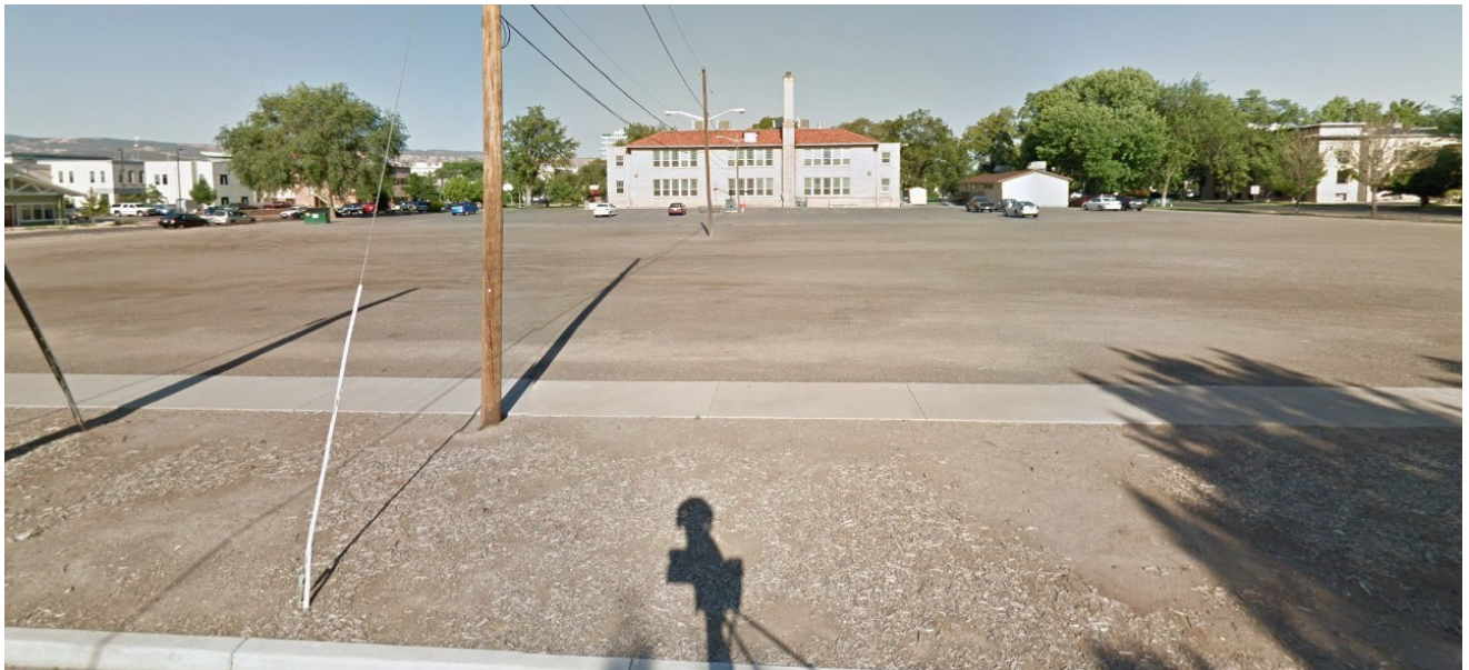
R-5 High School Site Looking West Platted Alley to be Vacated is Undeveloped but Building was Constructed Upon Right-of-Way
