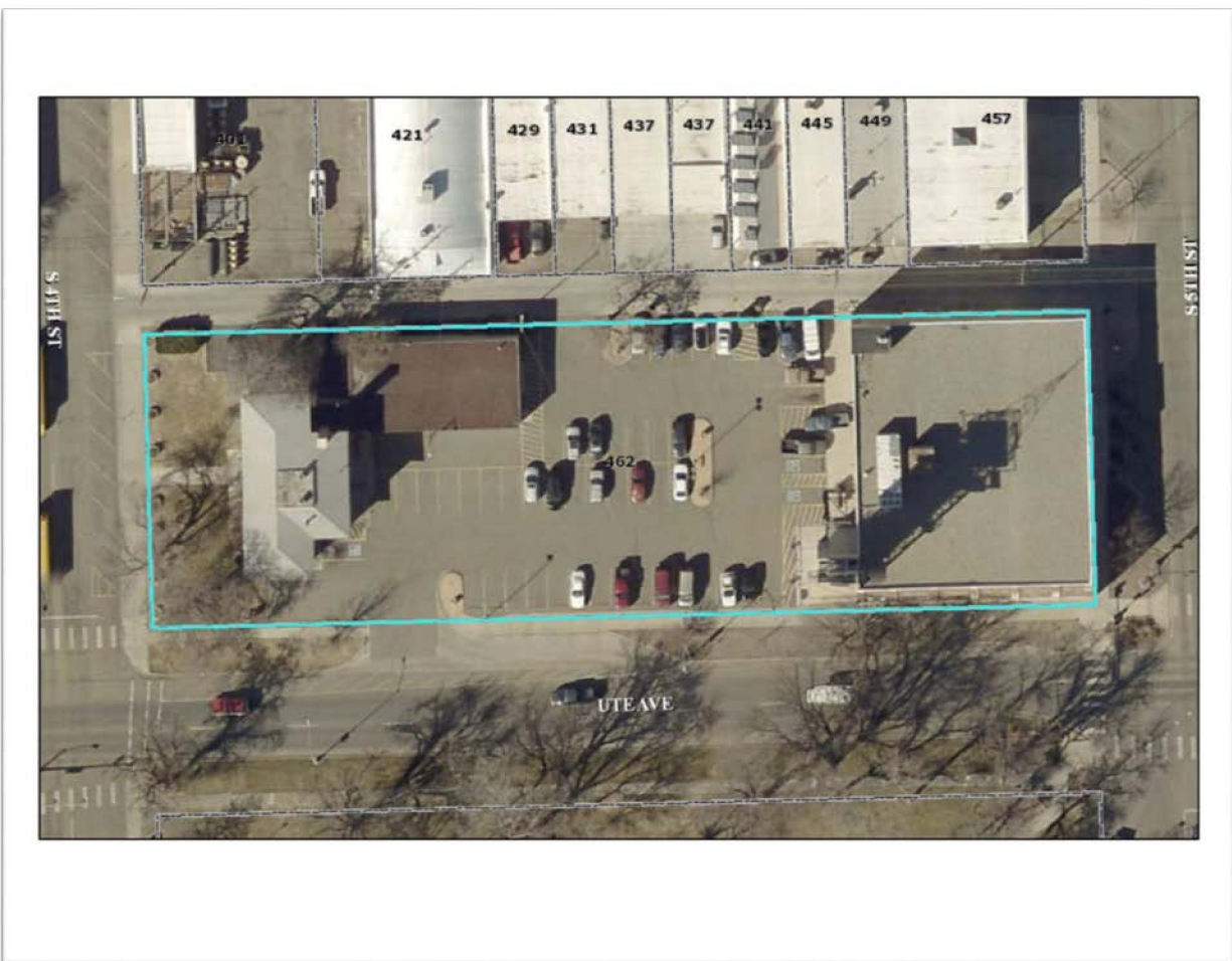
Figure 1 Existing Site and Buildings
