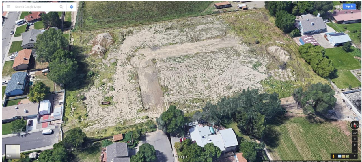
Overhead view of property from Redwing Lane
