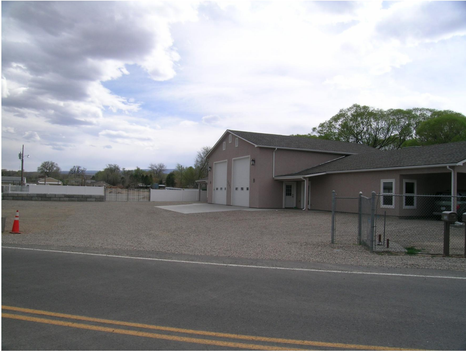
2723 Highway 50 - View from Hwy 50 Frontage Road looking south
