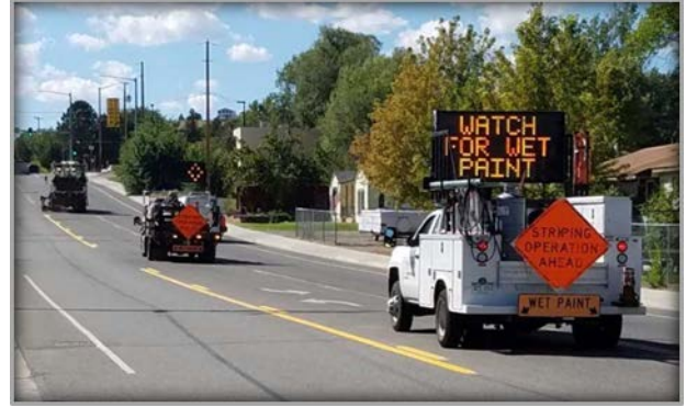
Street Striping Operation
