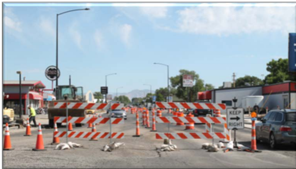
1 ST Street Reconstruction Project
