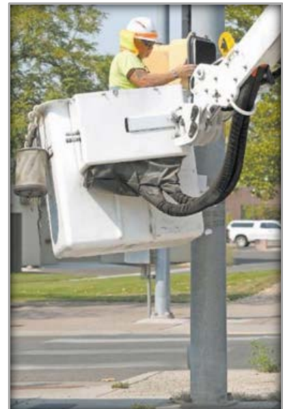
Signal Repair Work
