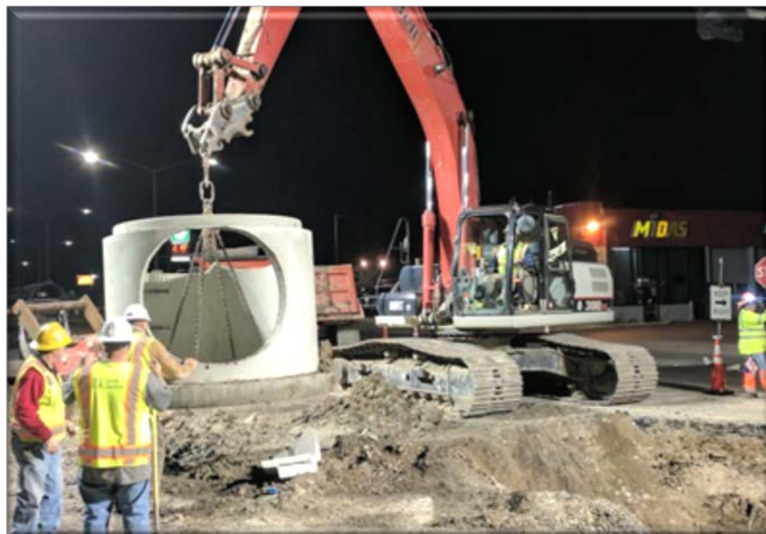
First Street Storm Drainage Improvements
