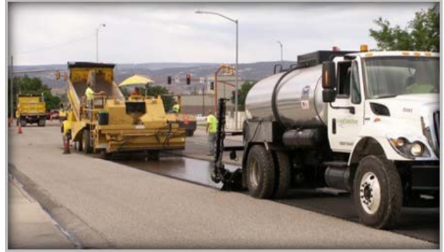
Street Overlay Work
