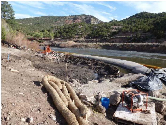
Example of dewatering.
