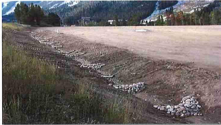
Photograph CD-1. Rock check dams in a roadside ditch. Photo courtesy of WWE.
