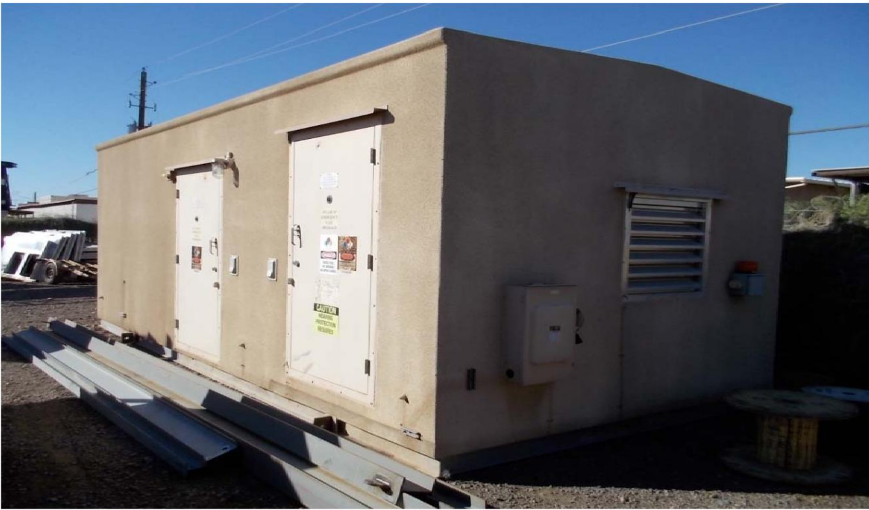
12 X26 Building that will be installed on site.
