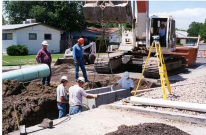
Orchard Avenue Major Storm Sewer Construction, Summer 1999
