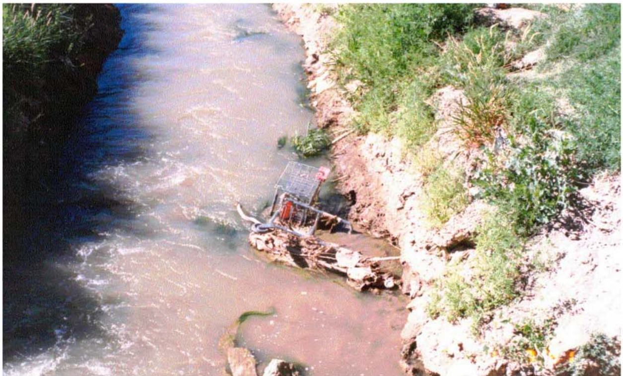
Figure 4. Example of Common Maintenance Needs
