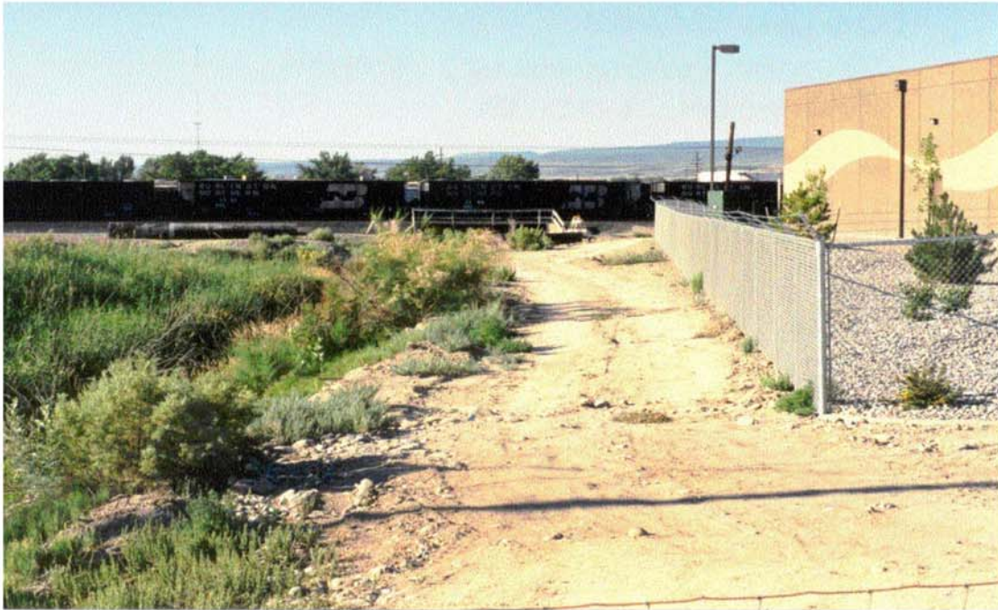
Figure 7. Hindrances to Maintenance Access
