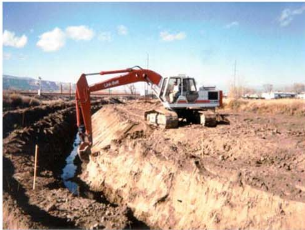
Ligrani Drain - Typical Open Drain Maintenance Activities
