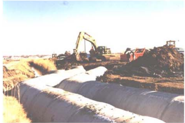
Capital Project - Ligrani Drain at Rimrock Market Place
