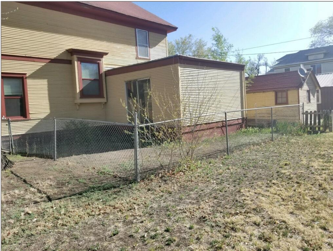
Existing Chain Link Fencing to be Replaced – Current Photo Provided by Applicant
