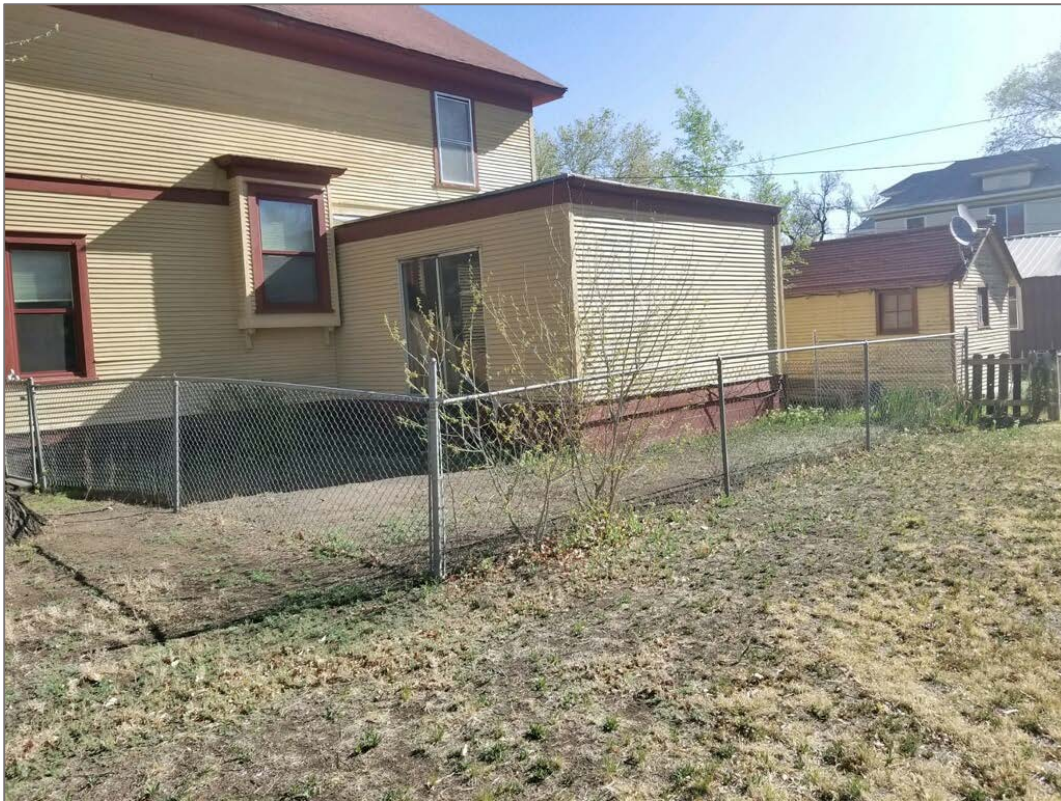
Existing Chain Link Fencing to be Replaced – Current Photo Provided by Applicant
