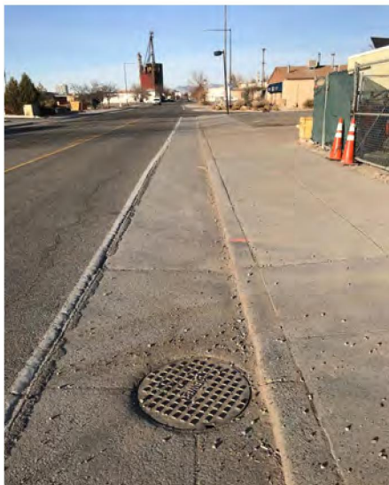
View of 7th Street and existing sewer in the sidewalk.
