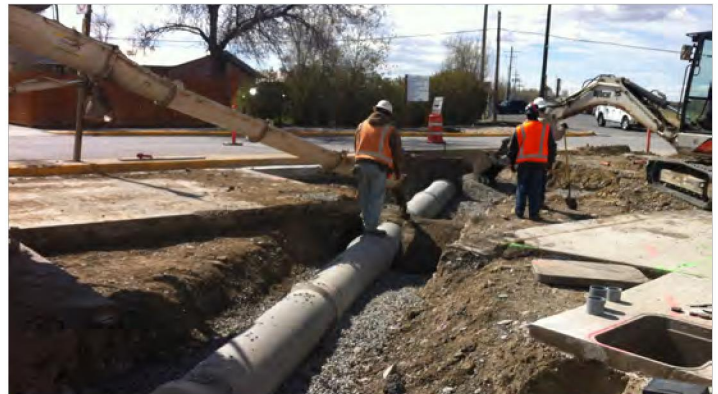
Installing new RCP storm sewer.
