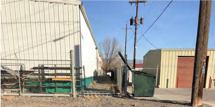
View of alley north of 3rd Avenue and potential utility impacts.
