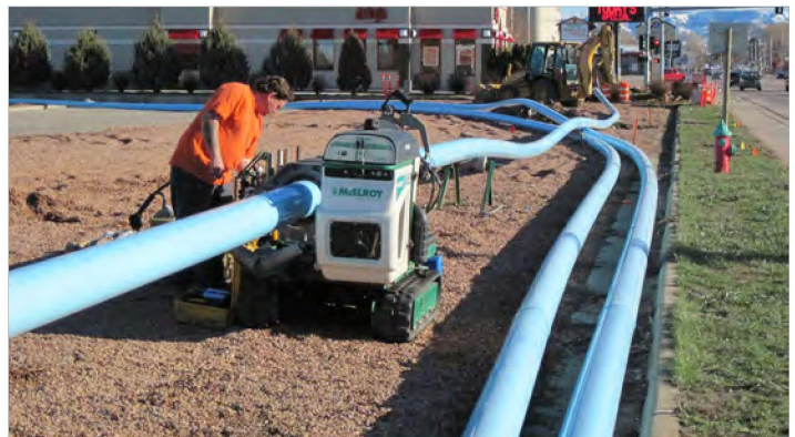
Fusing together C900 PVC water main for trenchless installation.
