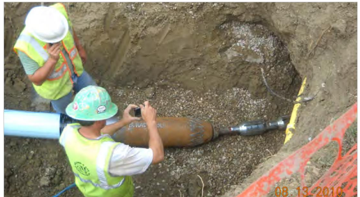
The pipe bursting head connected to the replacement PVC pipe.
