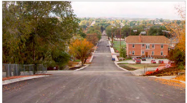
Completed 6th Street with its new pavement and curb and gutter.
