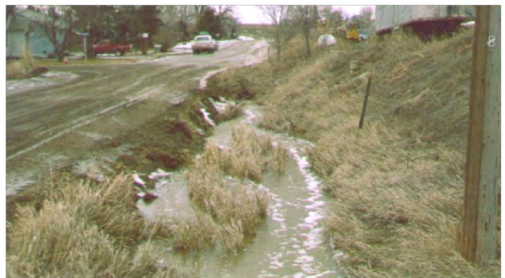
Prior to the improvements, storm drainage was poorly established and included ditches.
