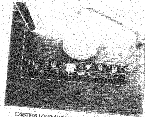
EXISTING LOGO AND LETTERS TO BE REPLACED WITH NEW W-28 SIGN EAST
