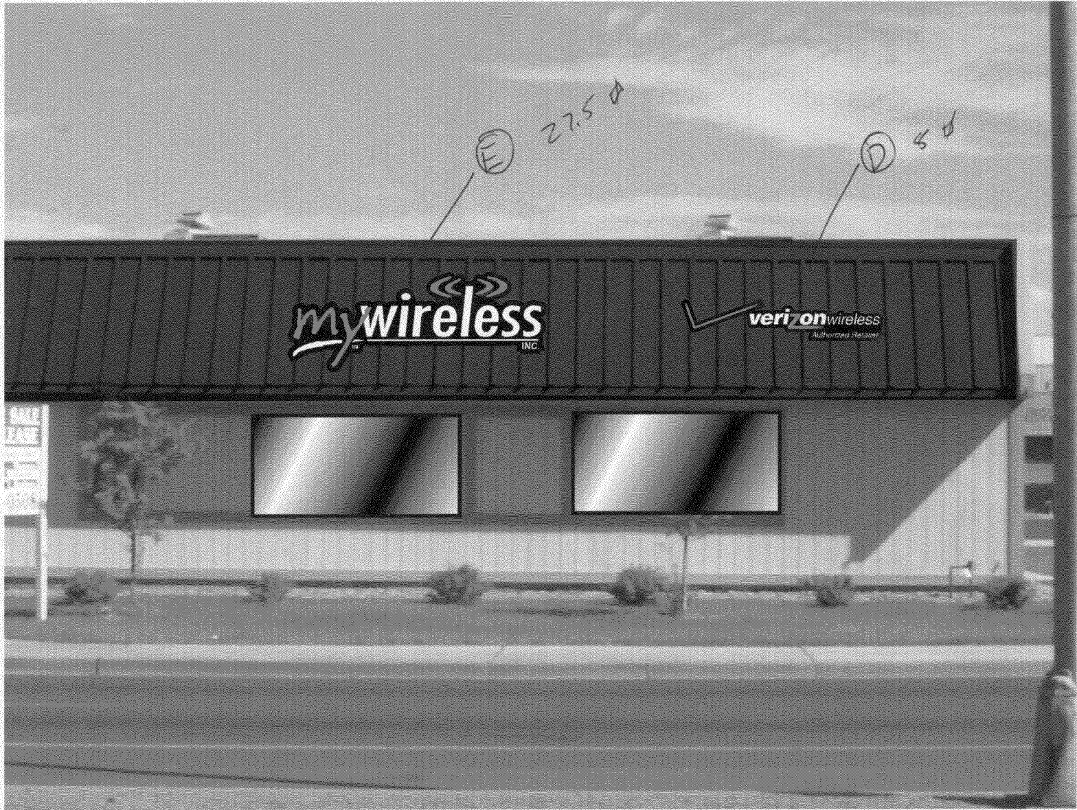
South Side of Building
