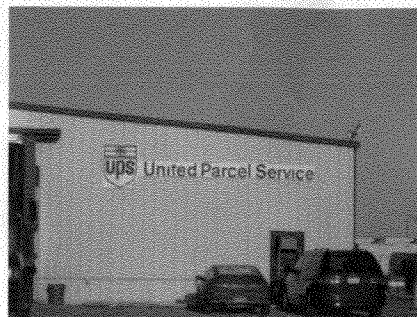
EXISTING BUILDING SIGNAGE TO BE REMOVED PER CORPORATE GUIDELINES
