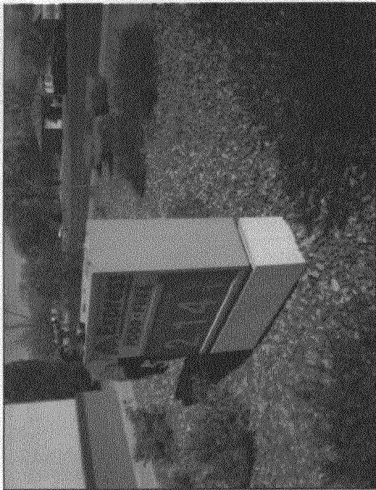
Remove & Discard Entire Monument Cabinets & Reveals Leave & Re-Use Existing Footing
