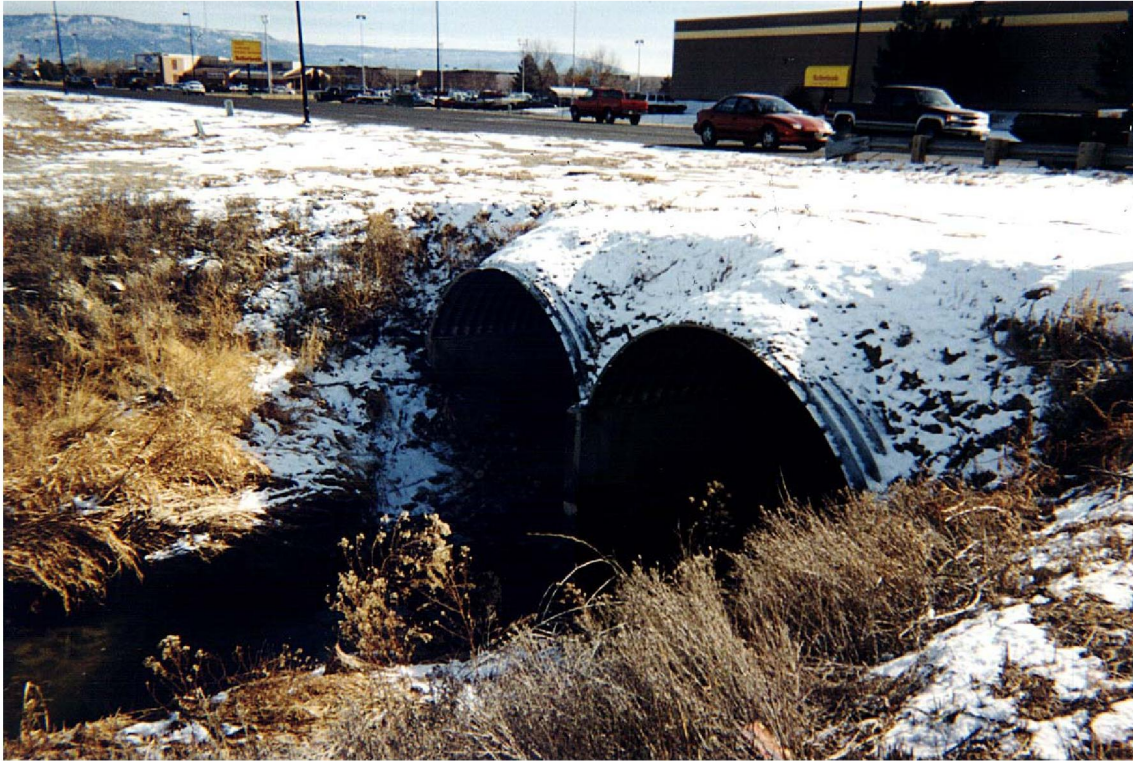
Existing Leach Creek drainage structure along 24 Road
