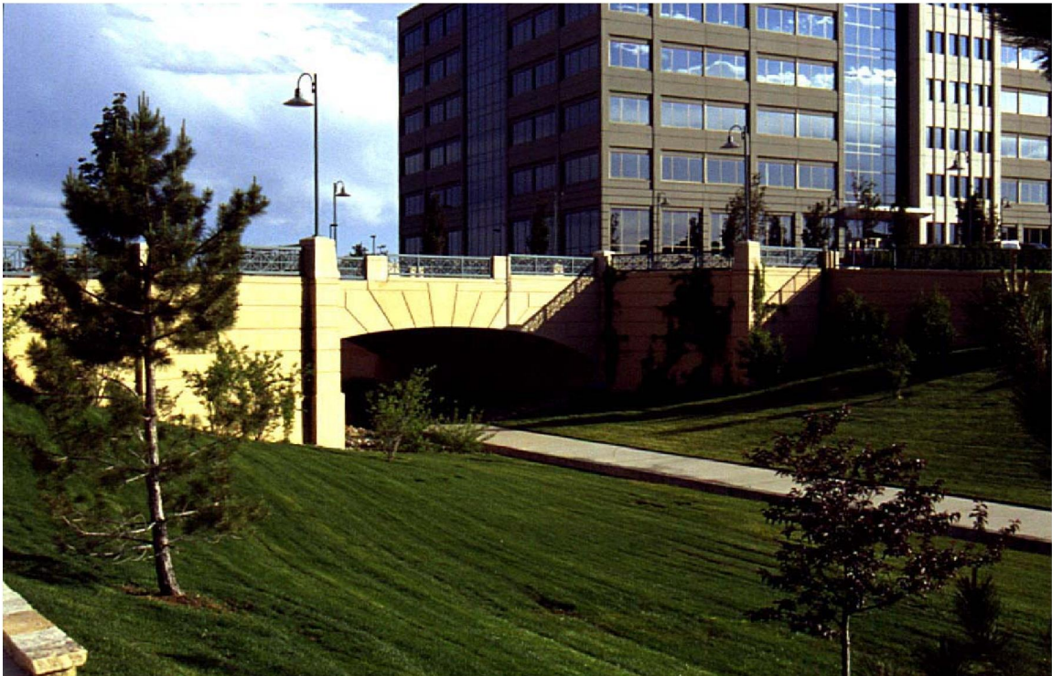
Open space incorporates drainage facility and amenities
