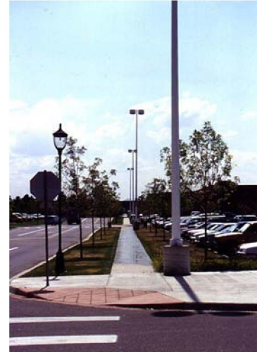
Pedestrian and street lighting in the right-of-way.
