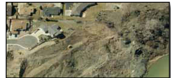
Figure 62: House sliding on Redlands bluff.
