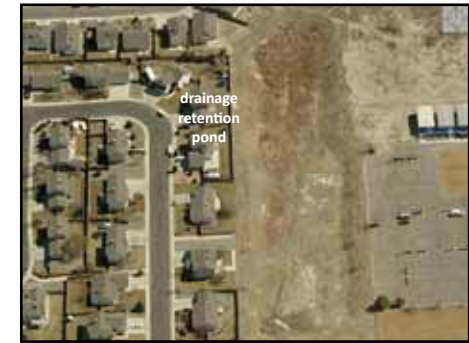
Figure 61: Detention pond at F Rd and 28 Rd.
