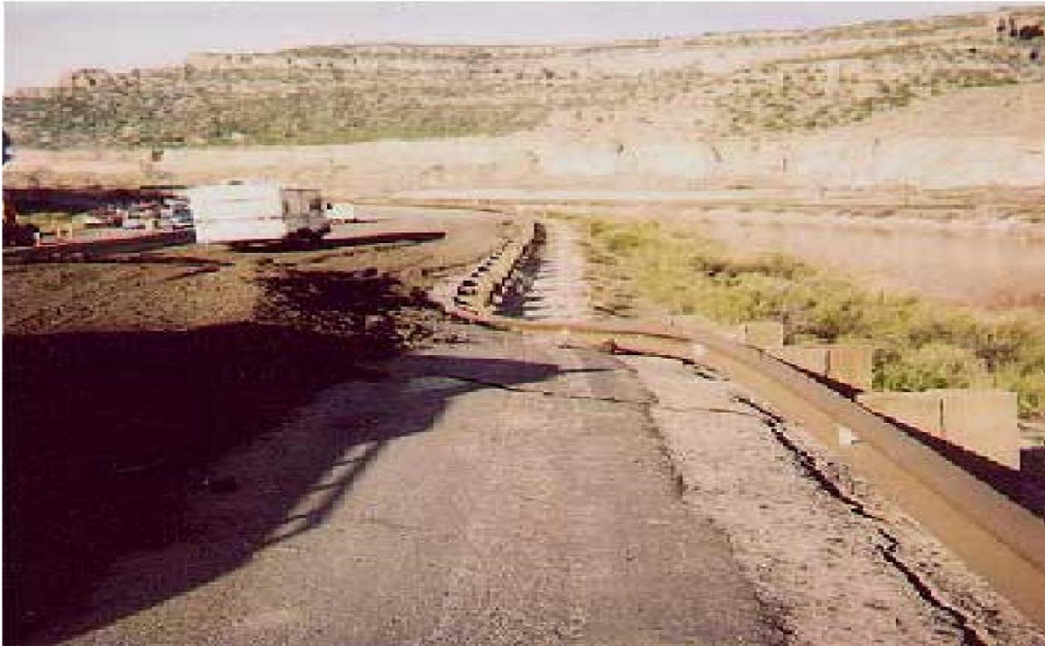
Figure 11: Photo of DeBeque Canyon Slide Area – Interstate 70
